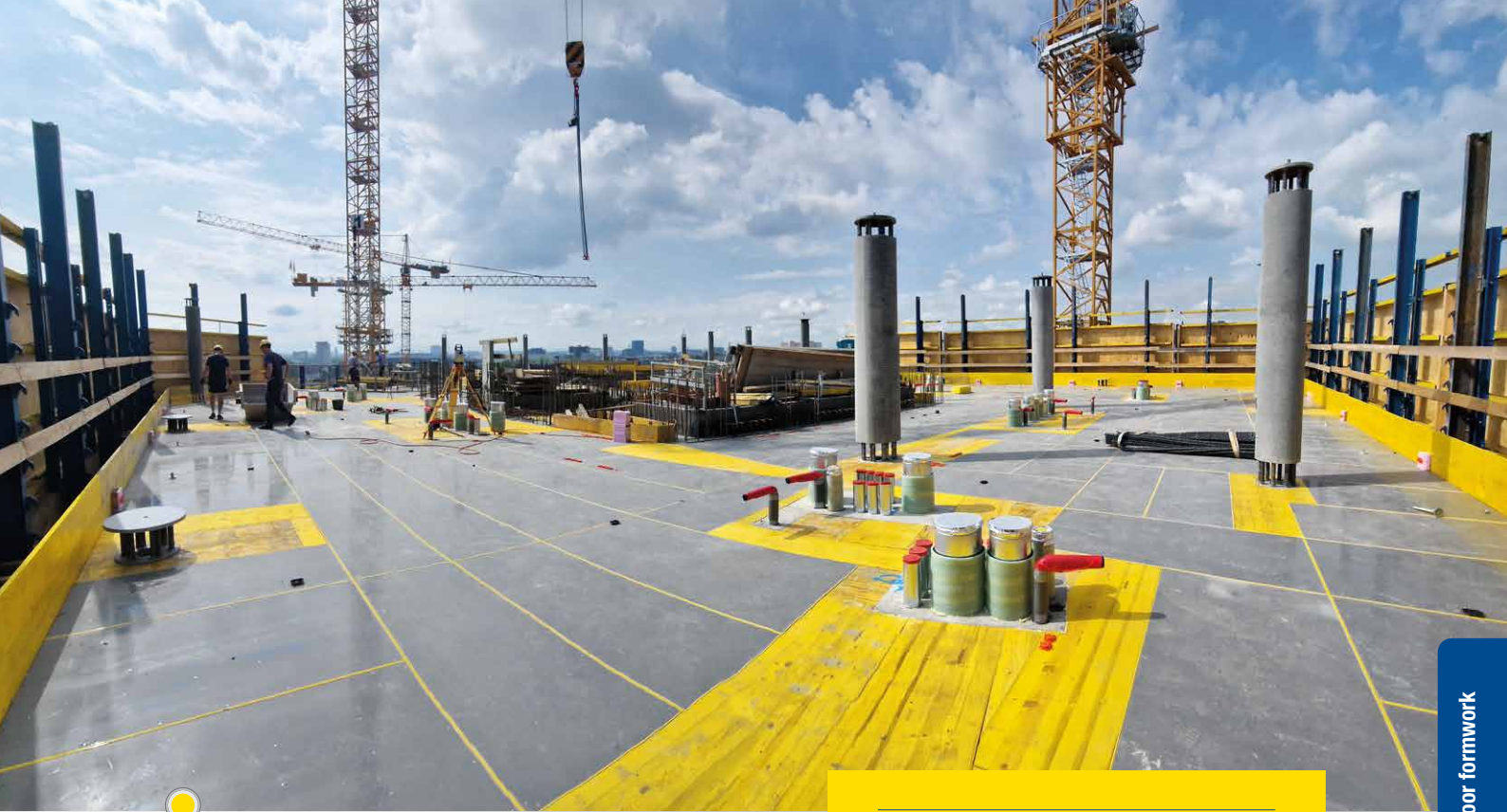
DokaXdek panel floor formwork in use
