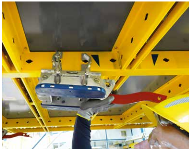
2. Swing the panel up into place
