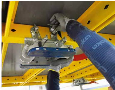
3. Insert pin to secure
