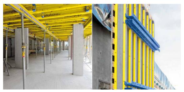
The high load capacity of the I tec 20 composite formwork beam means that fewer system components are needed. This saves on equipment and speeds up the construction workflow.
