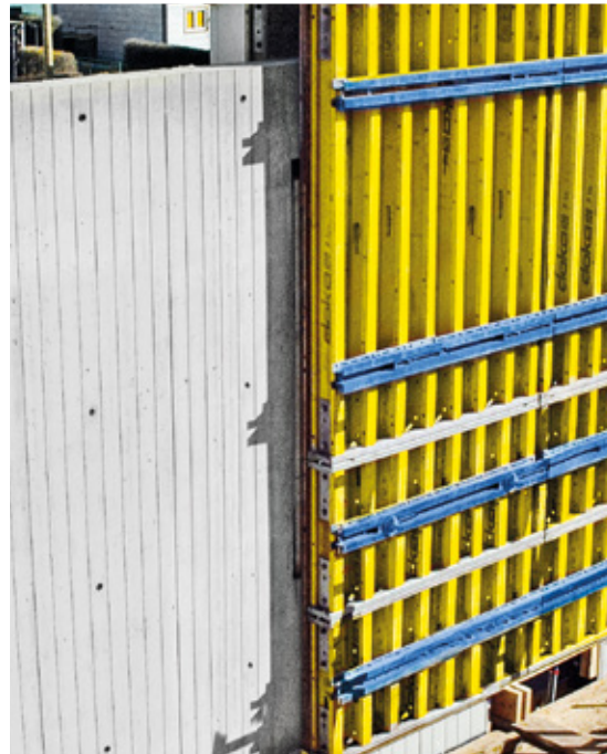
Outstanding fair-faced concrete quality by using Doka-Trenn, on structured surfaces.
