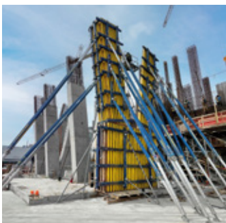
Tall walls & columns
