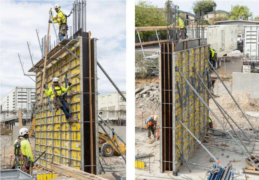
The Frami Xlife complete formwork system is ideal for shear walls. It's quick to assemble with few connections and ties, and also incorporates light clamps.
