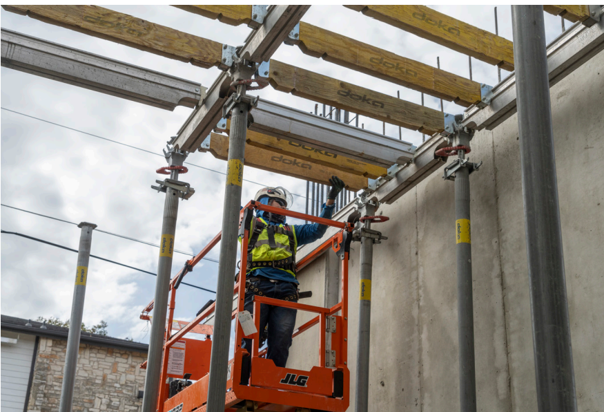
The SuperDek's drop head design provides superior stability while facilitating faster cycling times while the large grid capabilities reduce shoring and reshoring tasks.
